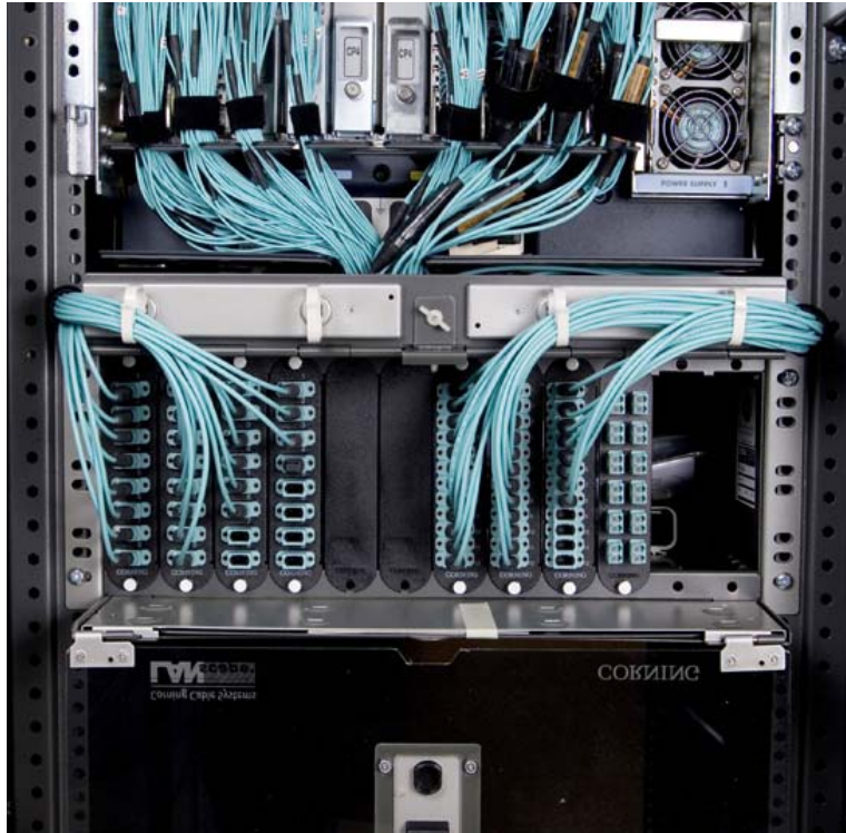
Figure 20. Cabling director blades with U-Space System
