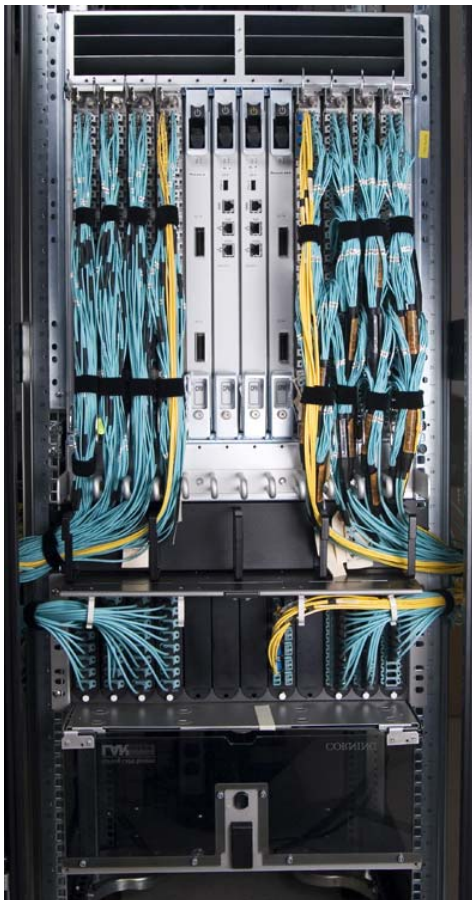
Figure 2. Corning Cable Systems cabling solutions on the Brocade DCX Backbone with 384 ports
